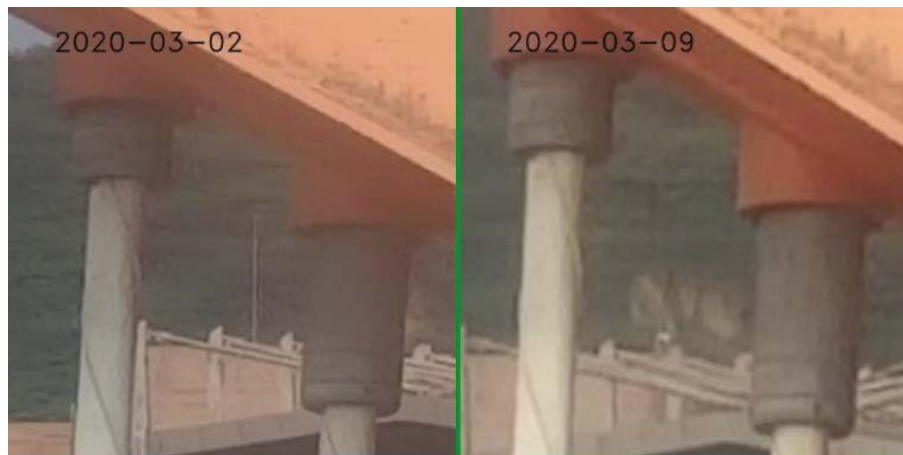
Figure 8 Bridge cable node 1 images between March 2 nd and March 9 th
