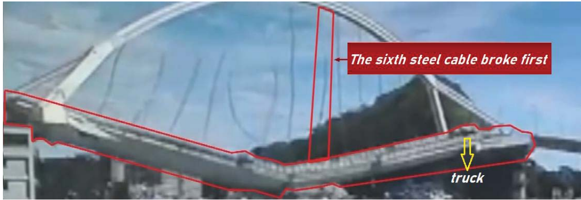
Figure 1 The sixth steel cable broke
