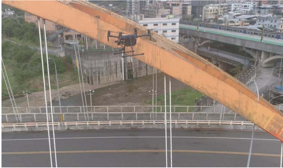
Figure 6 Camera drone take picture from bridge node
